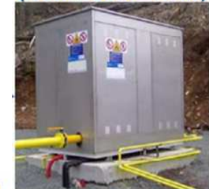
Pressure reduction (from 200 to 4 bar)
