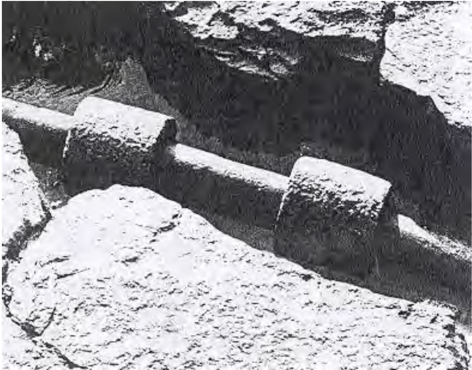
Fig. 3.22. The archaic hybrid solution of lead-pipes and stone-collars, in the Artemision of Ephesos (P. von Zabern, p.180)
